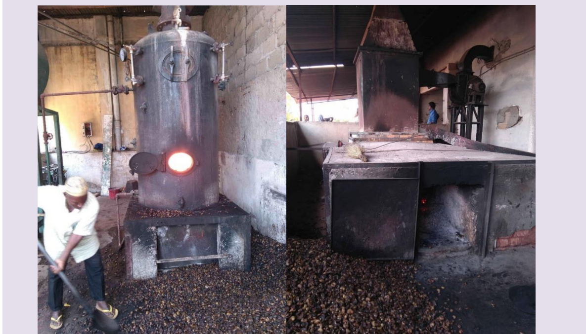
Figure 39. The pyrolysis oven can feed vertical boilers (on the left, Caju Ilha) and dryers (on the right, Mocaju).
