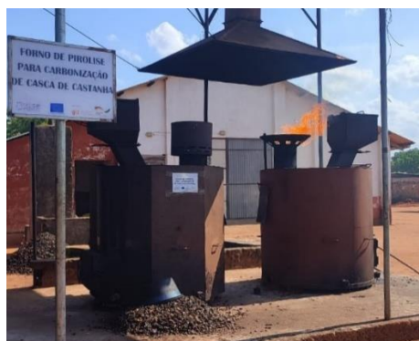
Carbonisation platform with two pyrolysis ovens
