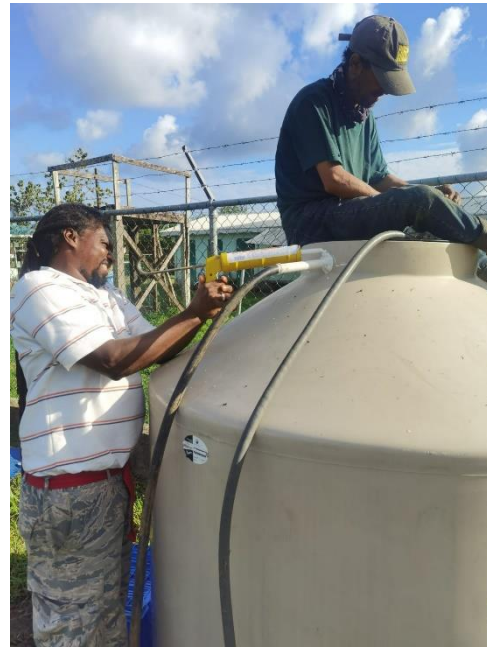
Figure 2: Revision of biodigester DEMO, fully working and producing 40 L of Biol fertilizer a day (left)
