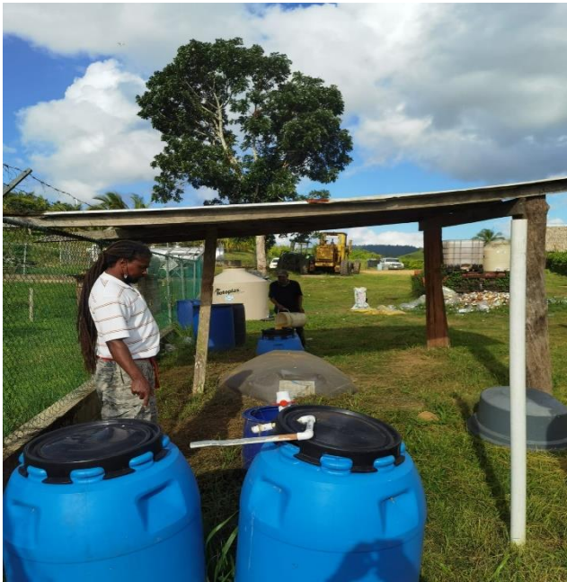
Figure 2: Revision of biodigester DEMO, fully working and producing 40 L of Biol fertilizer a day (left)
