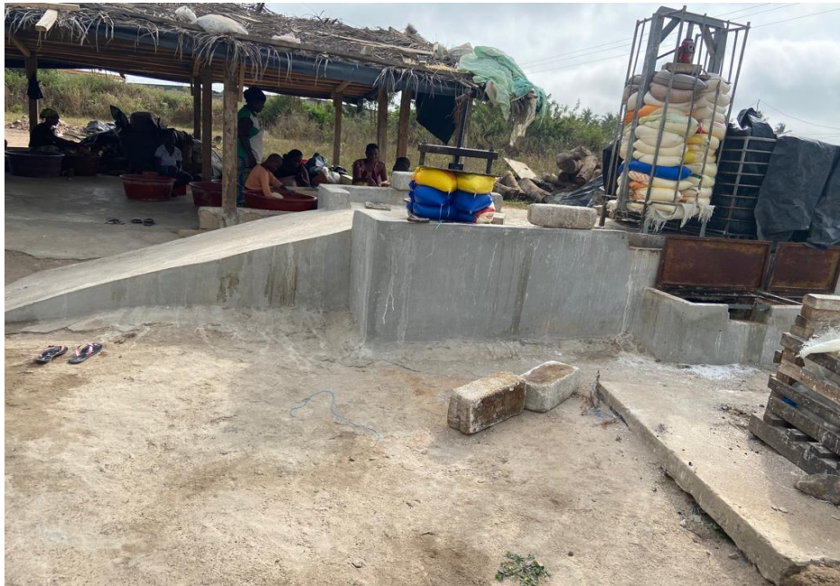
Figure 18: plateforme de pressage
