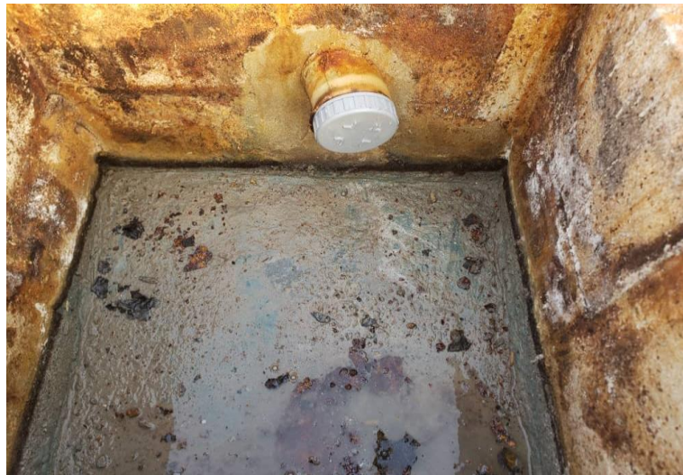
Figure 6: installation du bouchon pvc
