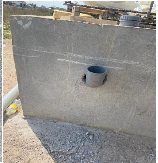
Figure 3: installation du coude pvc
