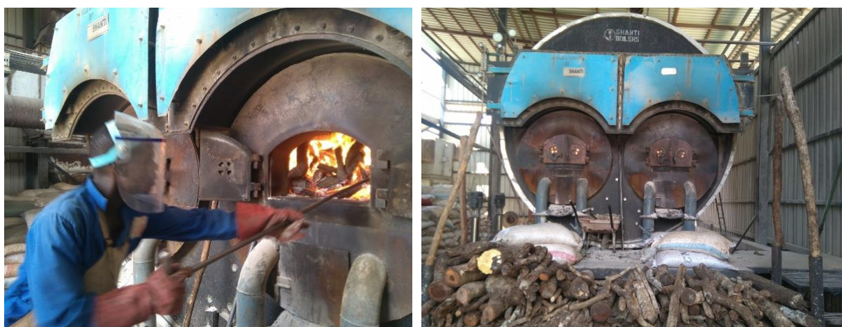
Figure 21. The factory boilers are manually fed with miombo wood logs
