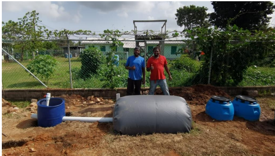
Biodigester V1 from VIOGAZ company, installed during second mission in TexStar farm
