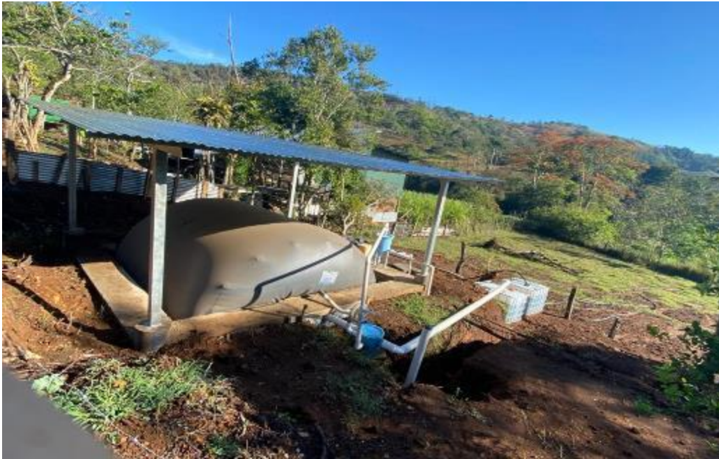
Viogaz digester model V25, with a liquid fertilizer system connected for good usage and IBC tanks on the right of the photo
